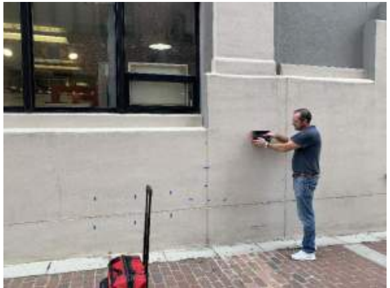
Fig 6: GPR Data collection through Exterior Wall
